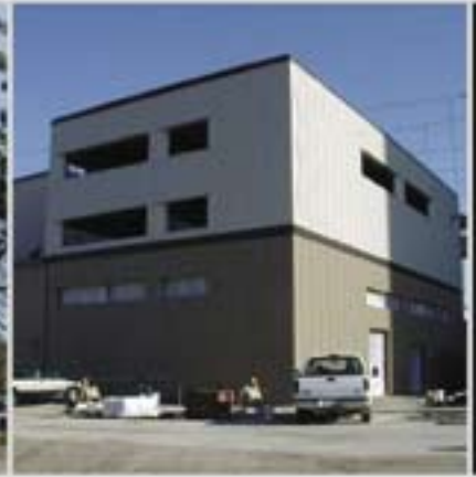
Ameren; Rush Island Plant: New 20,000 Square-Foot Administration Building
